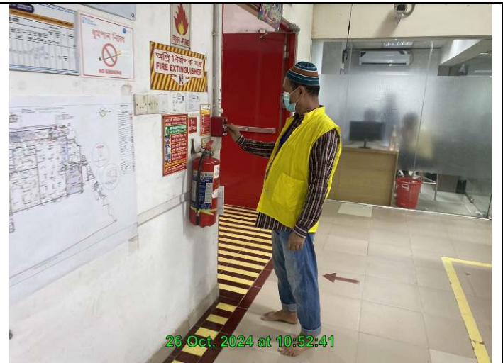
Fire alarm call point live testing
