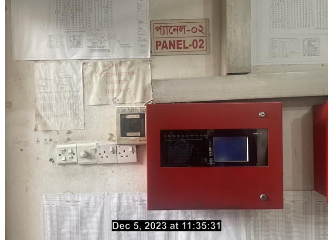
NC # 3.4.3 (d): Automatic fire detection disconnected
