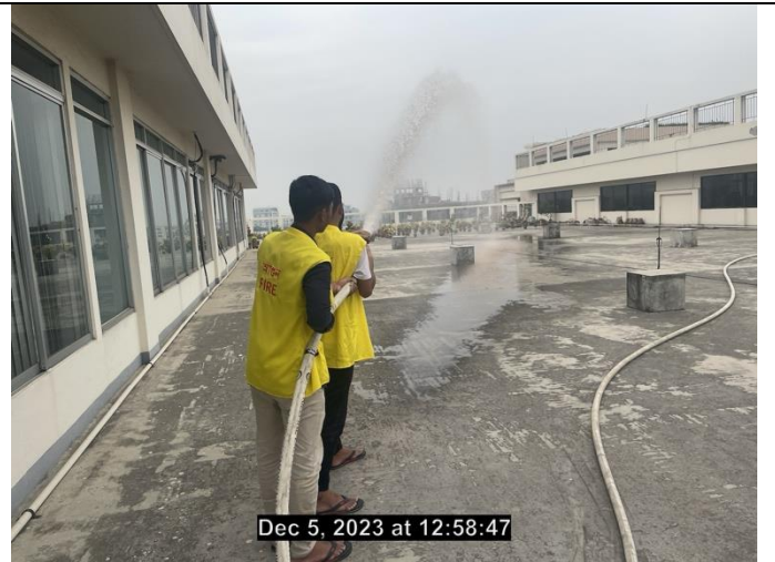
Fire hose live testing during the audit
