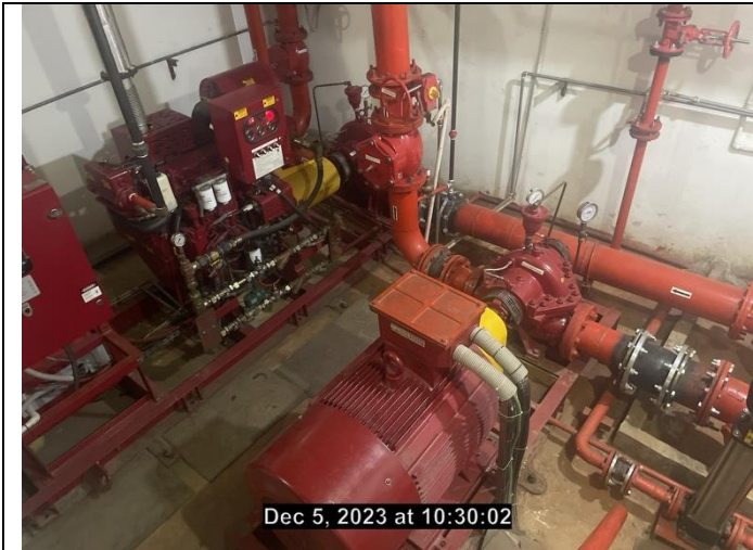
Fire hydrant pump house
