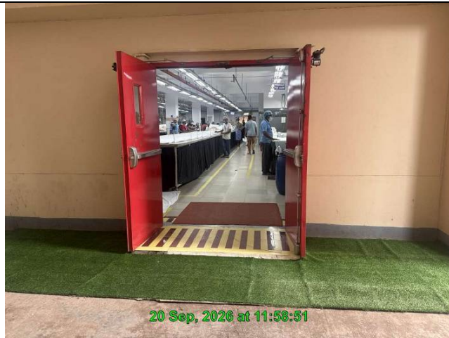
Exit door – Outward view
